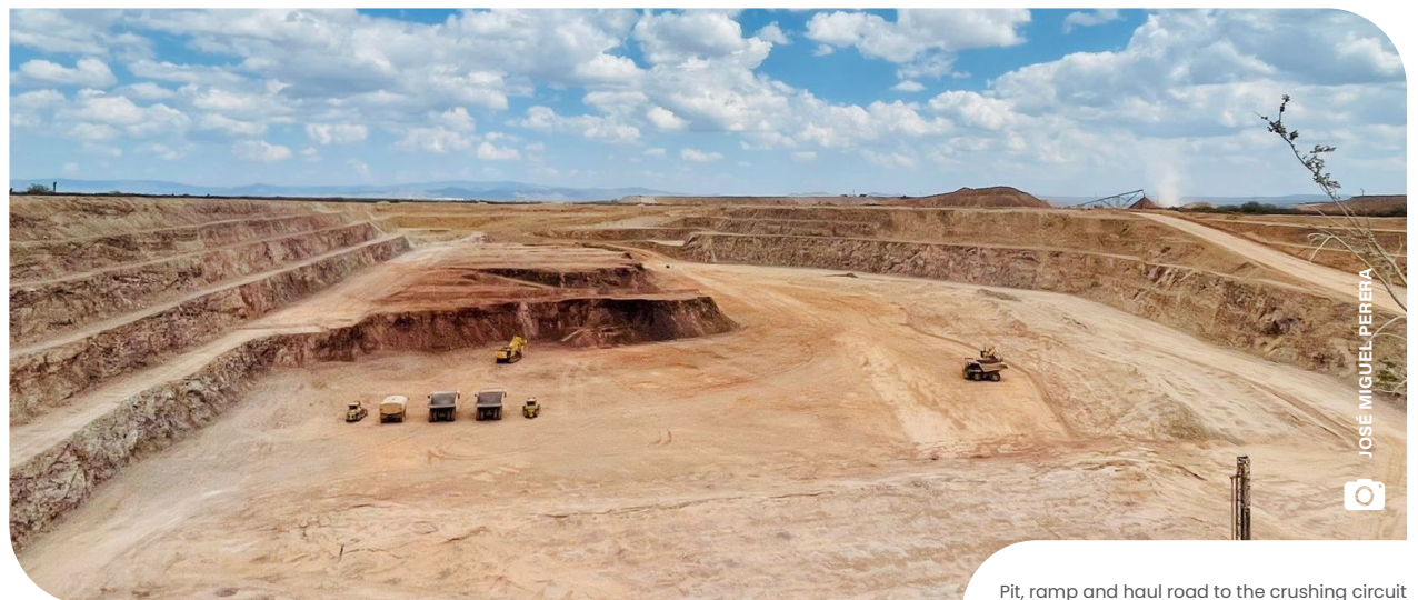
Pit, ramp and haul road to the crushing circuit
